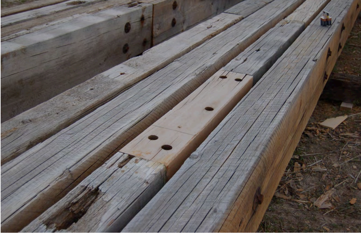
Figure 90: A dutchman repair.
