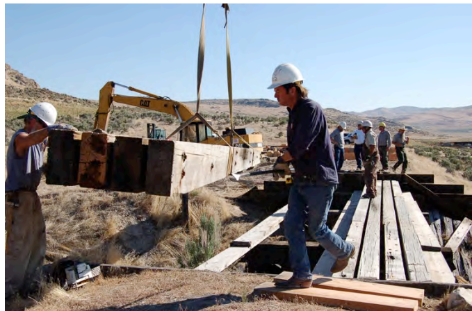
Figure 37: Lowering the second stringer assembly onto the trestle.
