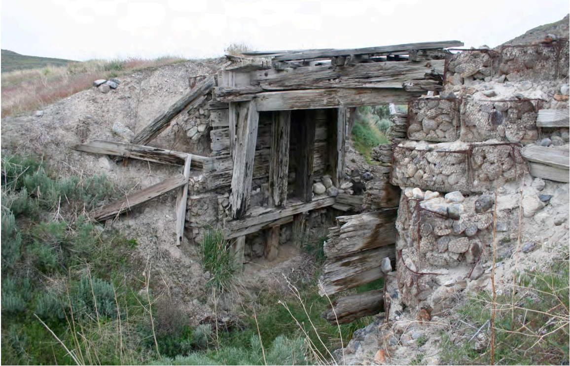
Figure 55: Trestle #1 before stabilization.
