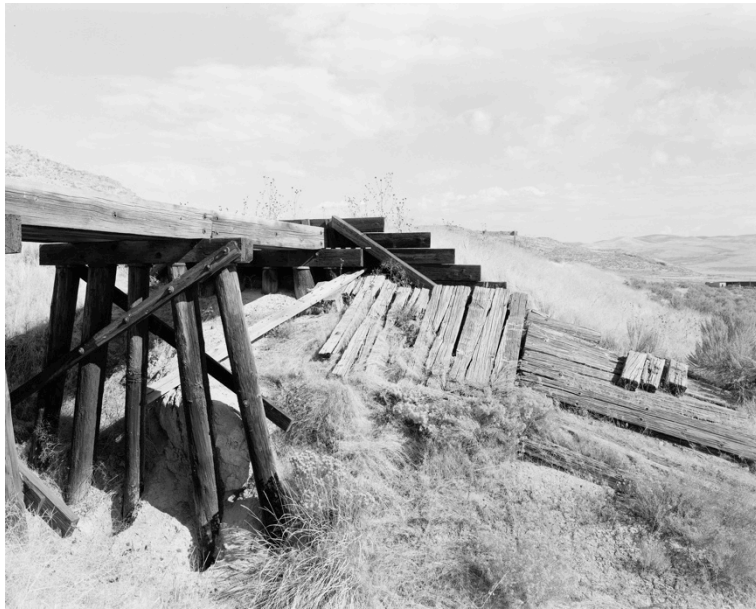
Figure 103: UT-64-7, Southern view of east bent and bulkhead.
