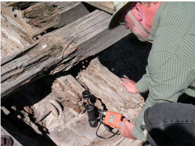
Figure 7: Determining the moisture content of a top strut, Trestle #1.
