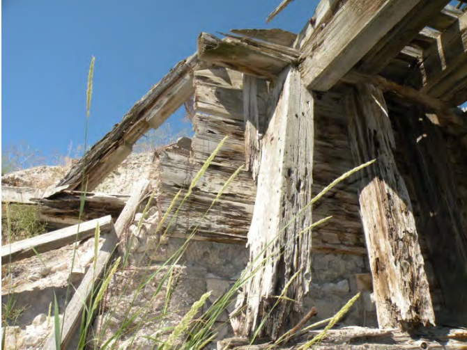
Figure 20: The southwest wing wall.
