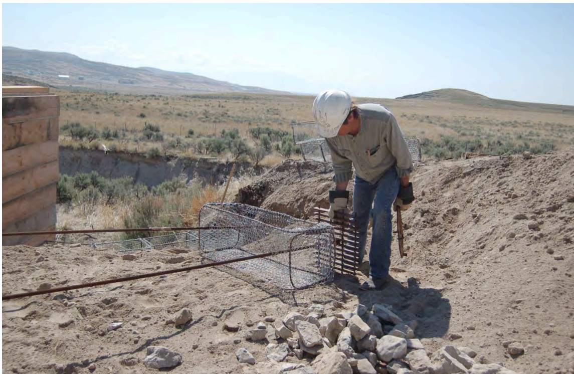
Figure 77: A second deadman was installed behind the northwest wing wall.
