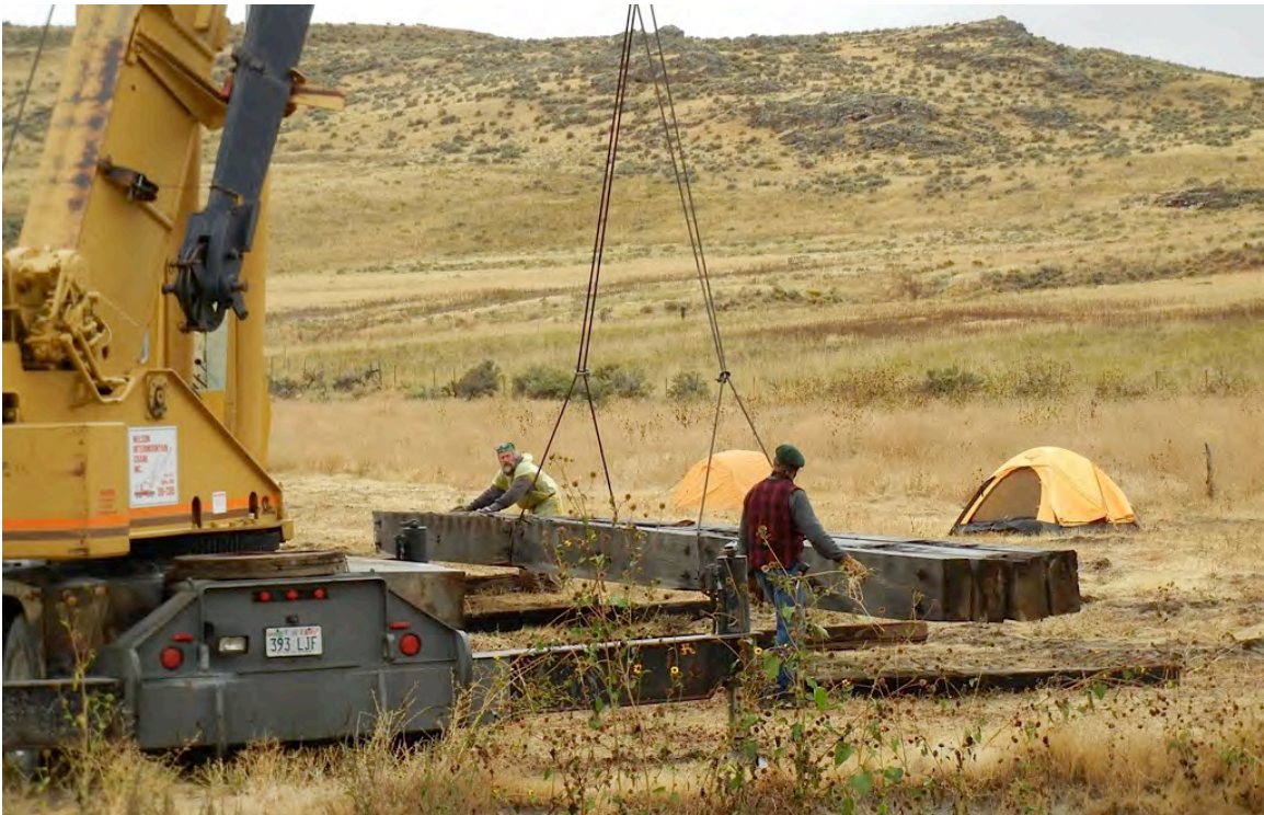
Figure 89: The assemblies were then set on timber beds for repair.
