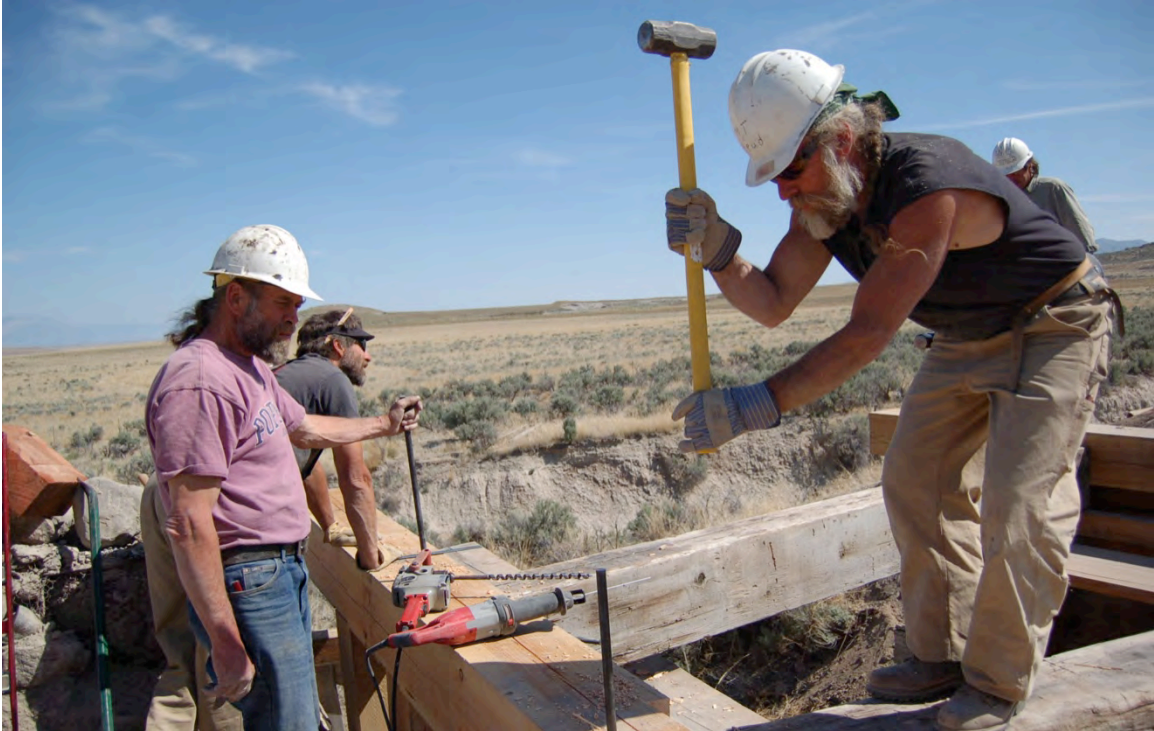
Figure 82: Driving drift pins through a pile cap into the piles below.
