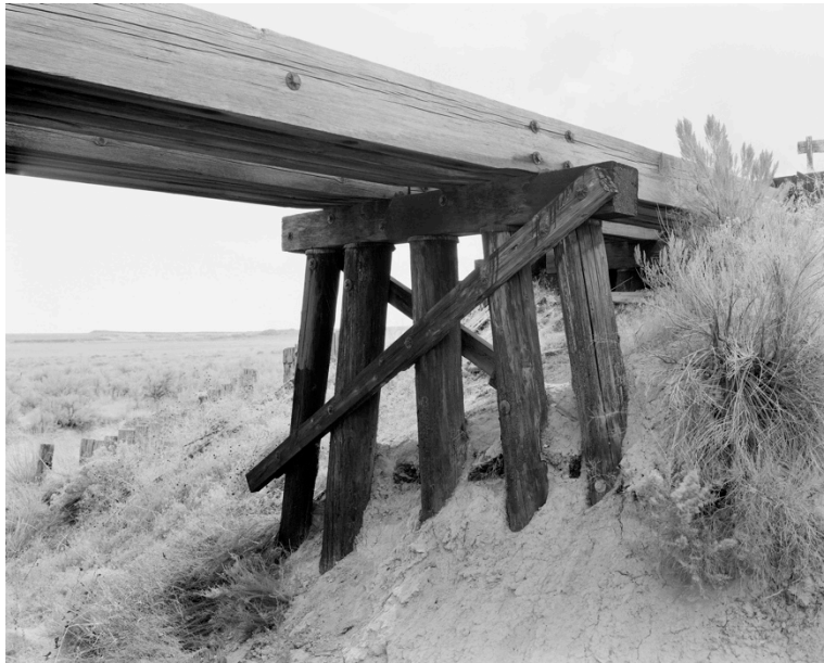
Figure 107: UT-64-11, Northern view of west bent.
