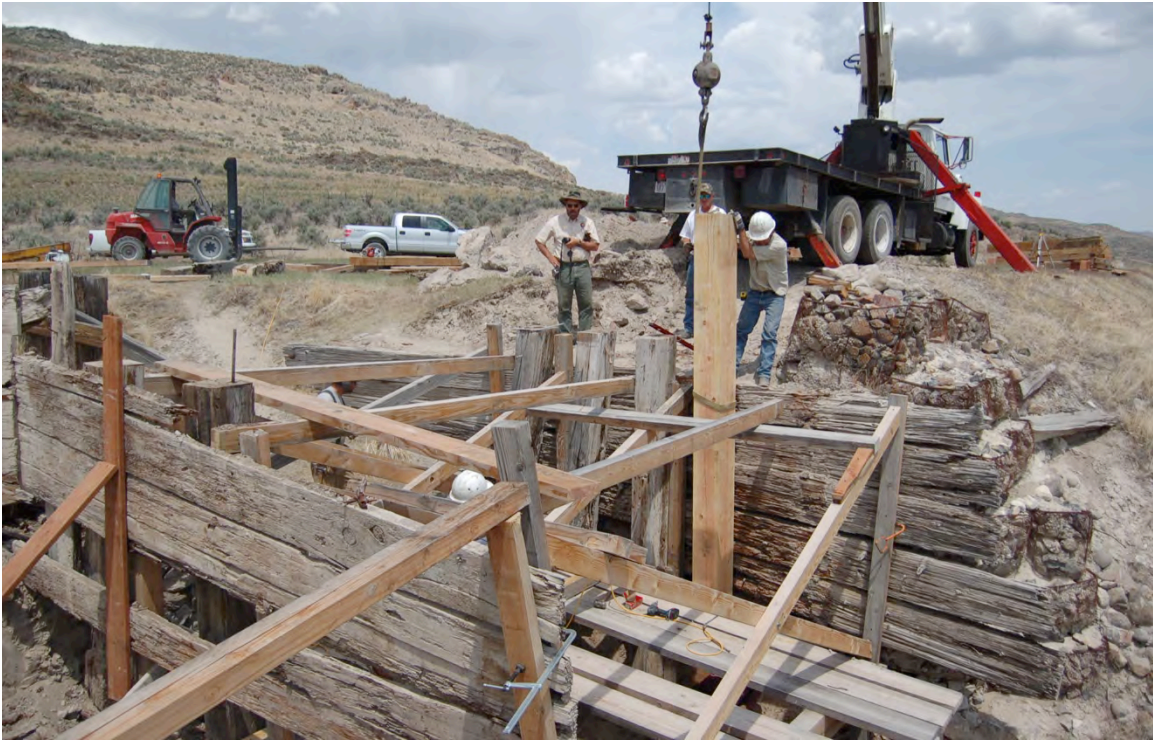
Figure 58: Lowering a replacement pile into position at the east bent.
