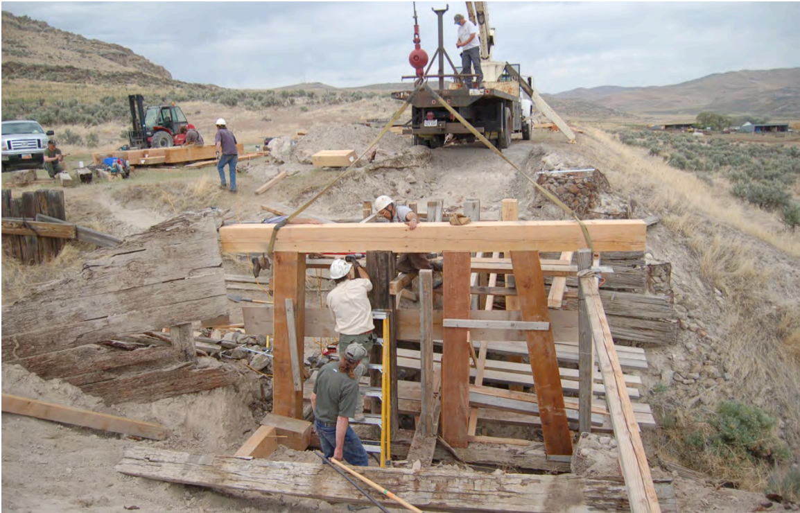
Figure 65: A replacement pile cap is positioned on the west bent.
