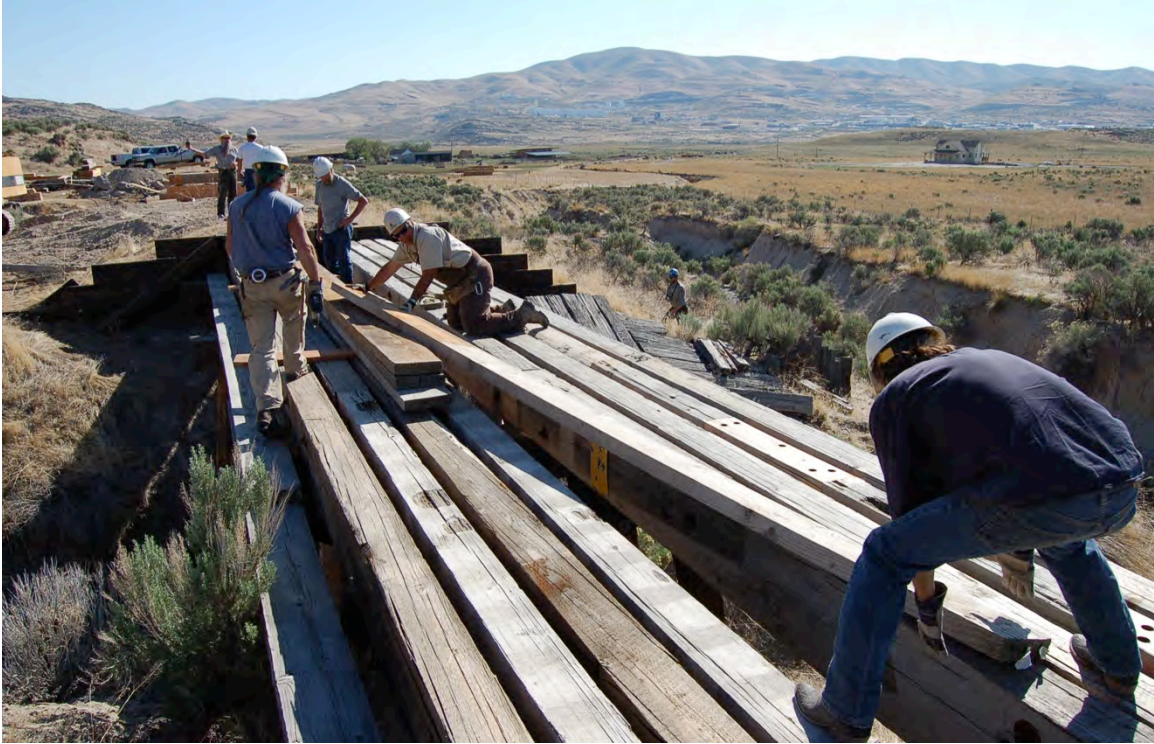
Figure 94: Removing the planking from around the stringers.
