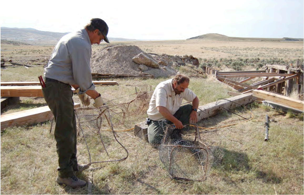
Figure 71: Gabion cages that could be salvaged were straightened and rewired.
