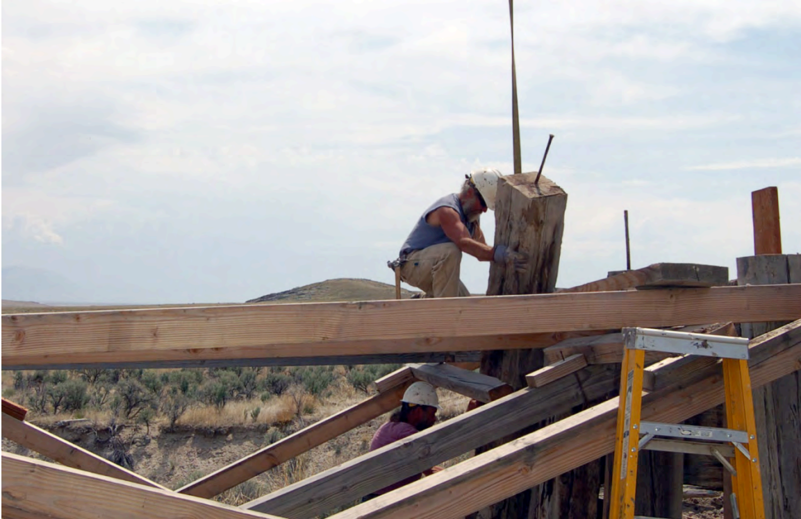
Figure 57: Removing an unsalvageable pile from the west bent.
