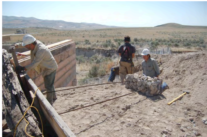
Figure 33: Tie-backs installed at the northwest wing wall.
