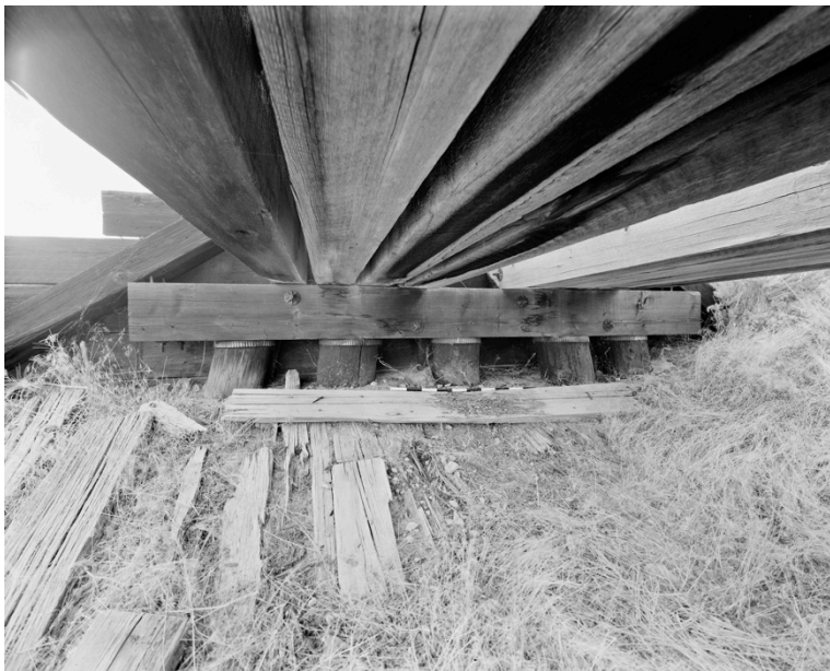
Figure 108: UT-64-12, West bulkhead.
