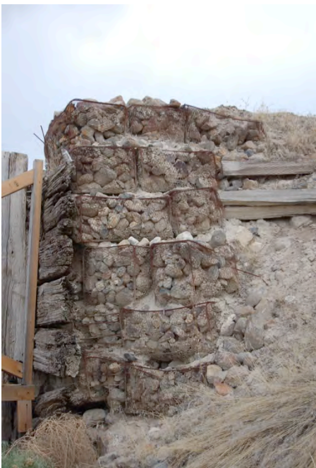
Figure 21: Gabions at the east bulkhead.
