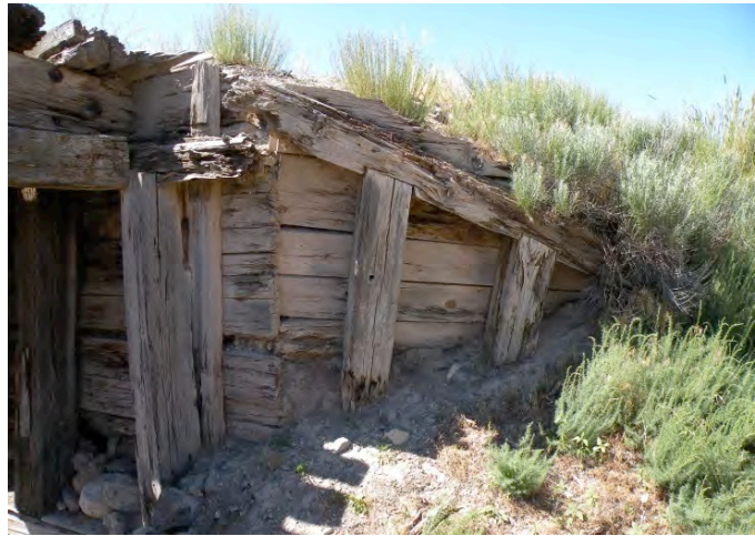
Figure 18: The northwest wing wall.
