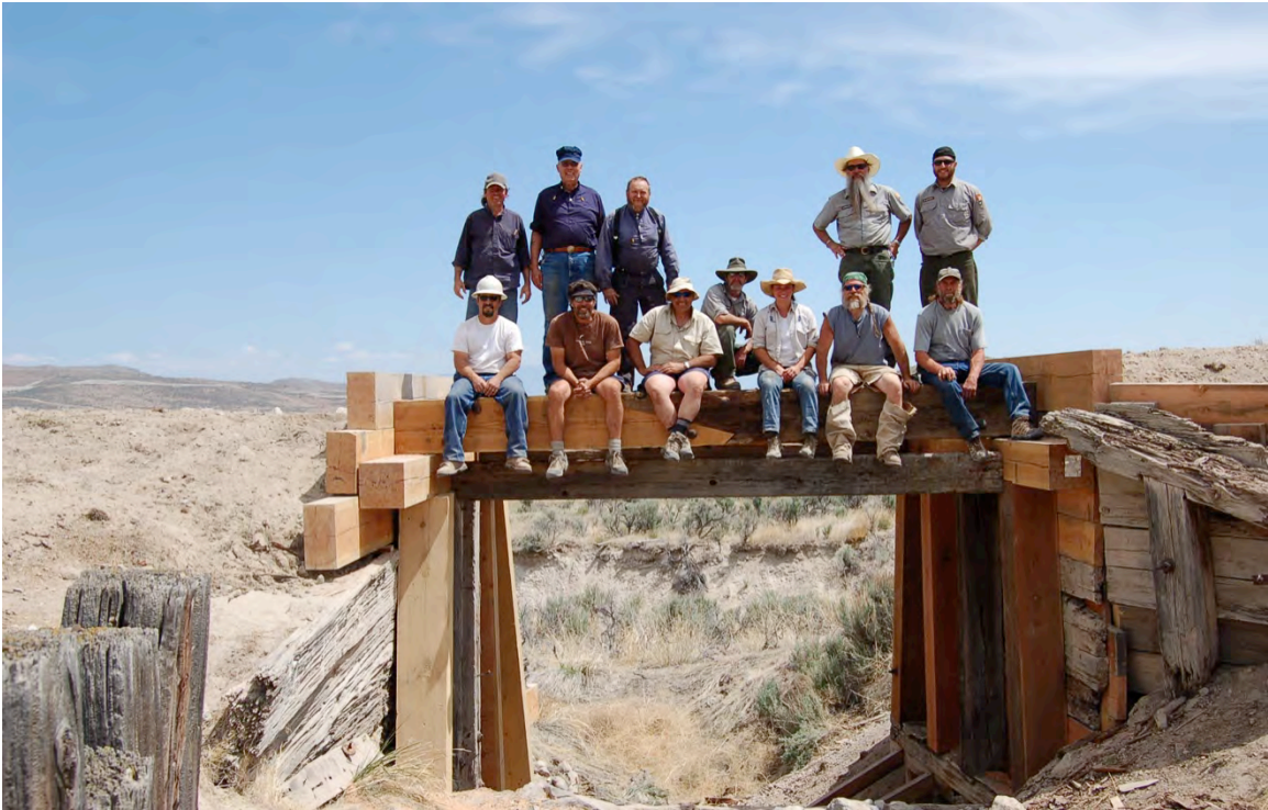
Figure 85: Trestle #1 after stabilization.
