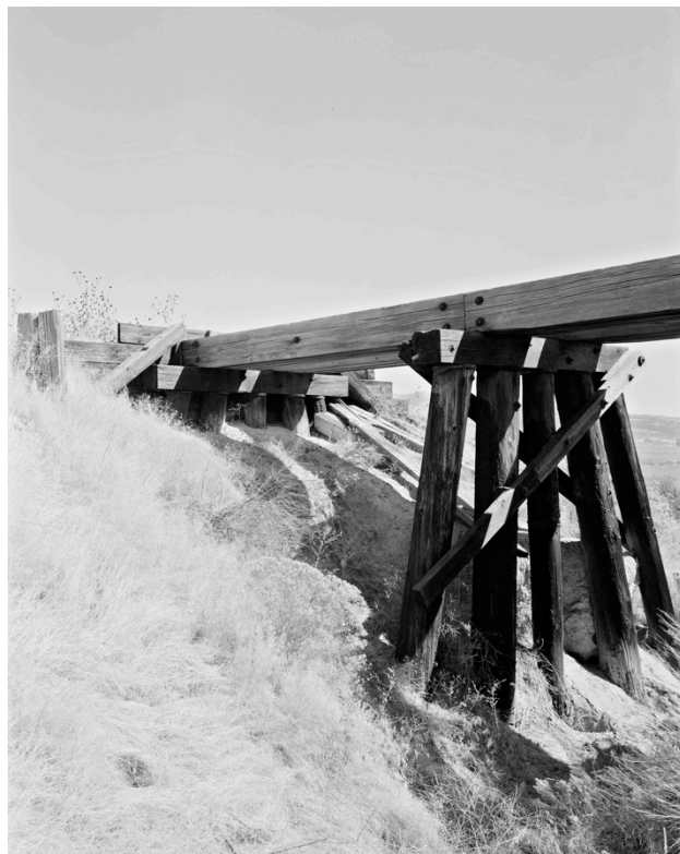
Figure 104: UT-64-8, Northern view of east bent and bulkhead.
