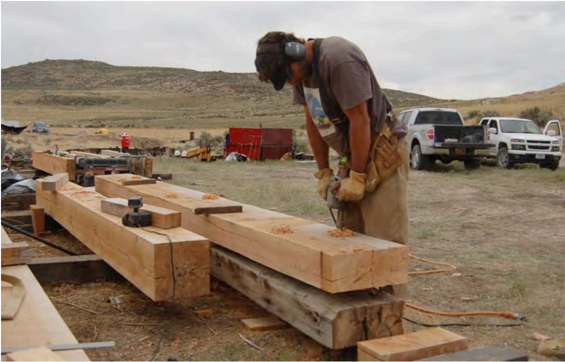
Figure 66: Drilling holes for the stringer hardware.
