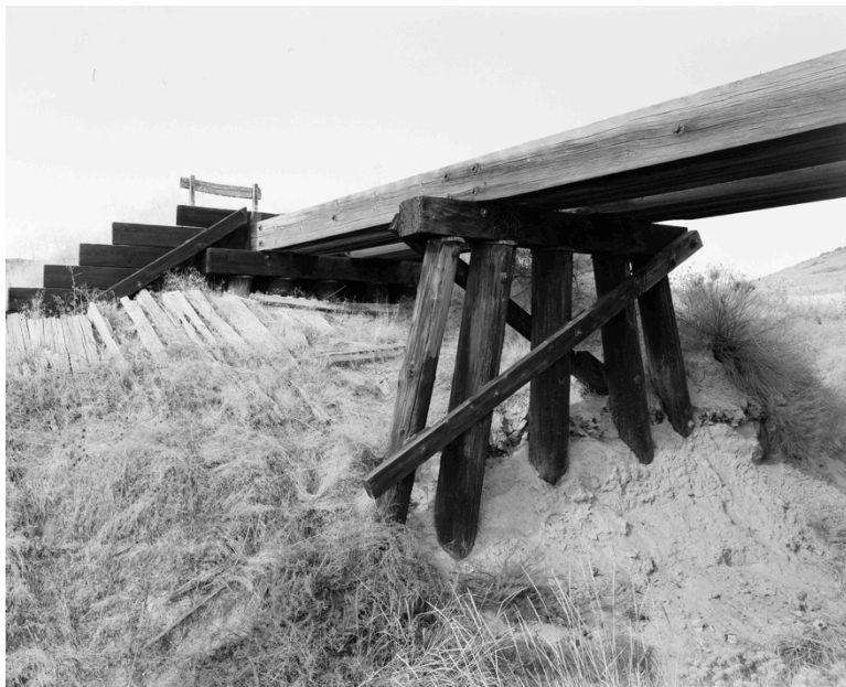
Figure 106: UT-64-10, Southern view of west bent and bulkhead.
