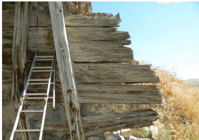
Figure 19: Southeast wing wall.
