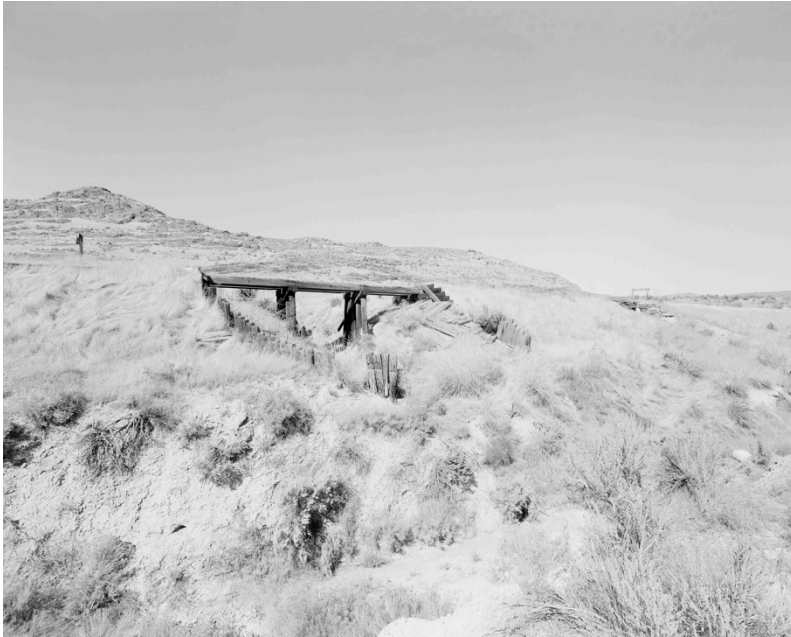
Figure 97: UT-64-1, General area of Trestle #2.
