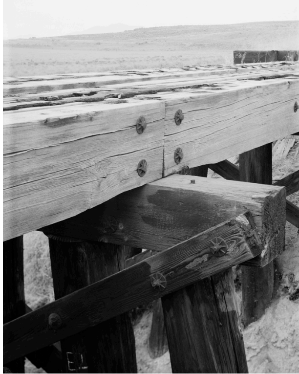
Figure 109: UT-64-13, Detail of stringers and pile cap.
