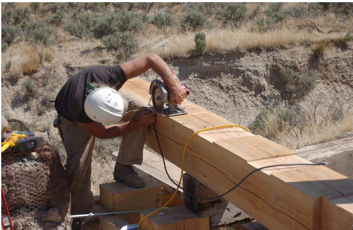
Figure 78: Rabbeting the pile cap for the east bent.
