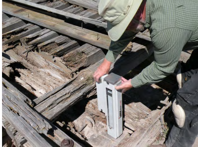
Figure 8: Using the resistance drill in a top strut, Trestle #1.
