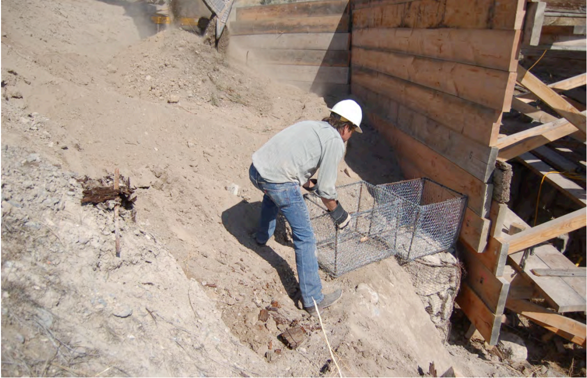
Figure 75: Gabions were replaced along the south slope behind the west bulkhead.
