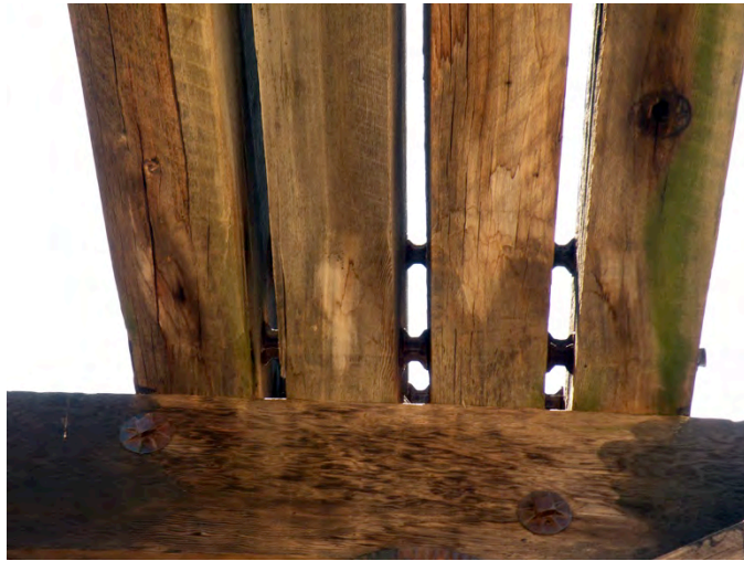
Figure 10: Clear wood stringers on Trestle #2 consistent with a high structural grade.
