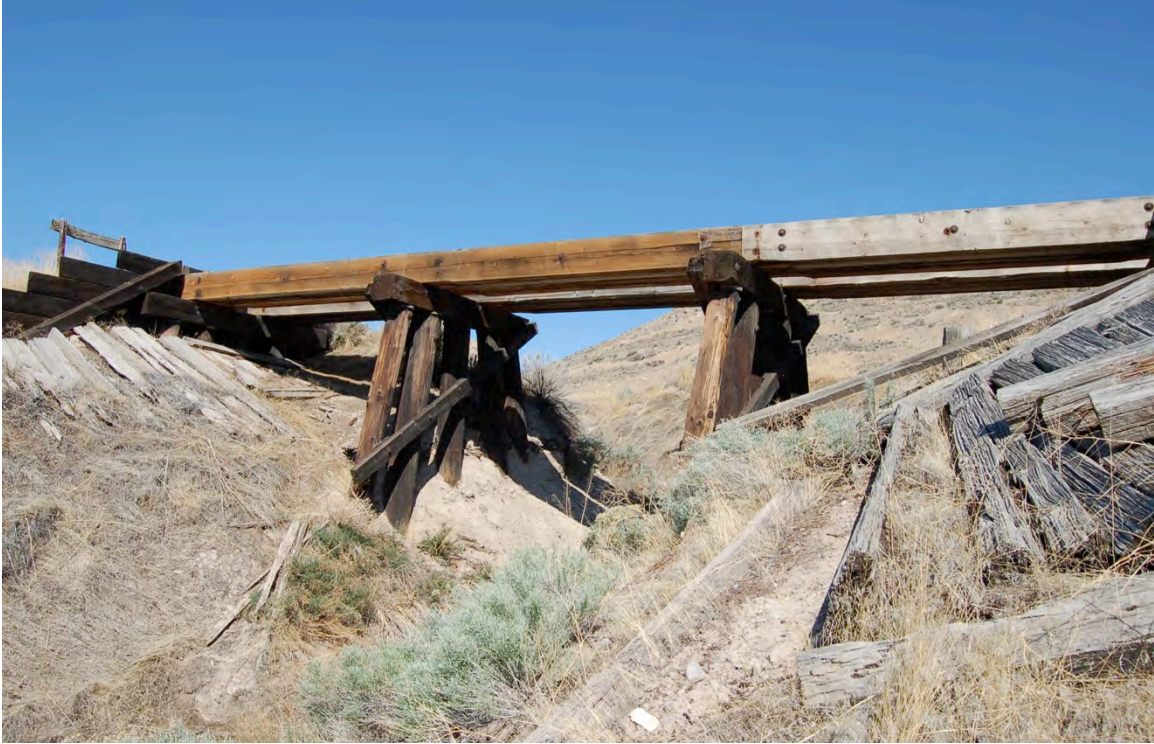
Figure 96: Trestle #2 after stabilization.
