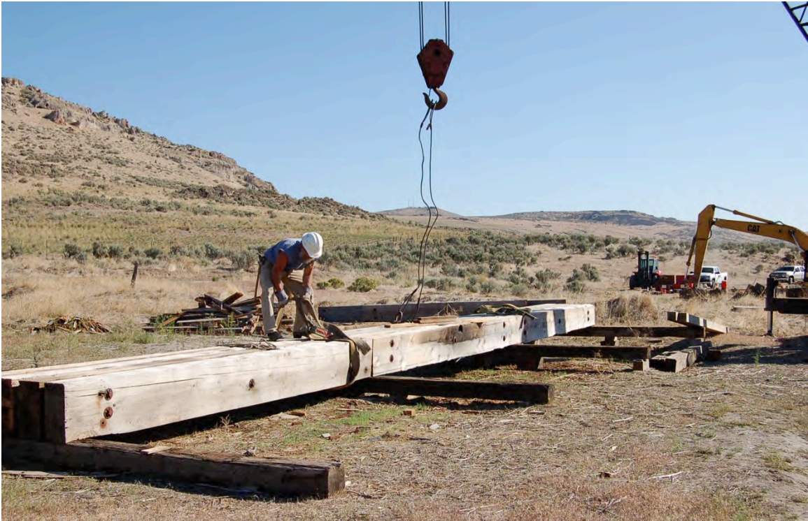
Figure 91: Rigging for the crane after repair and reassembly.
