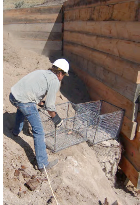
Figure 32: Setting new gabions at the south end of the west bulkhead.
