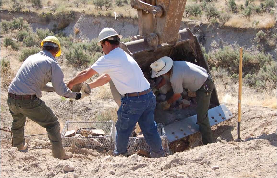
Figure 76: Filling the gabions with stone salvaged from the originals.
