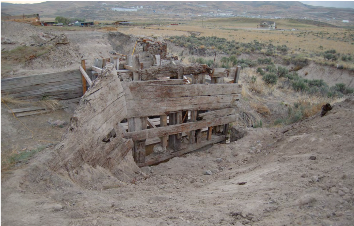
Figure 56: The west bulkhead after excavation. Note the extreme deterioration of the bulkhead planking.
