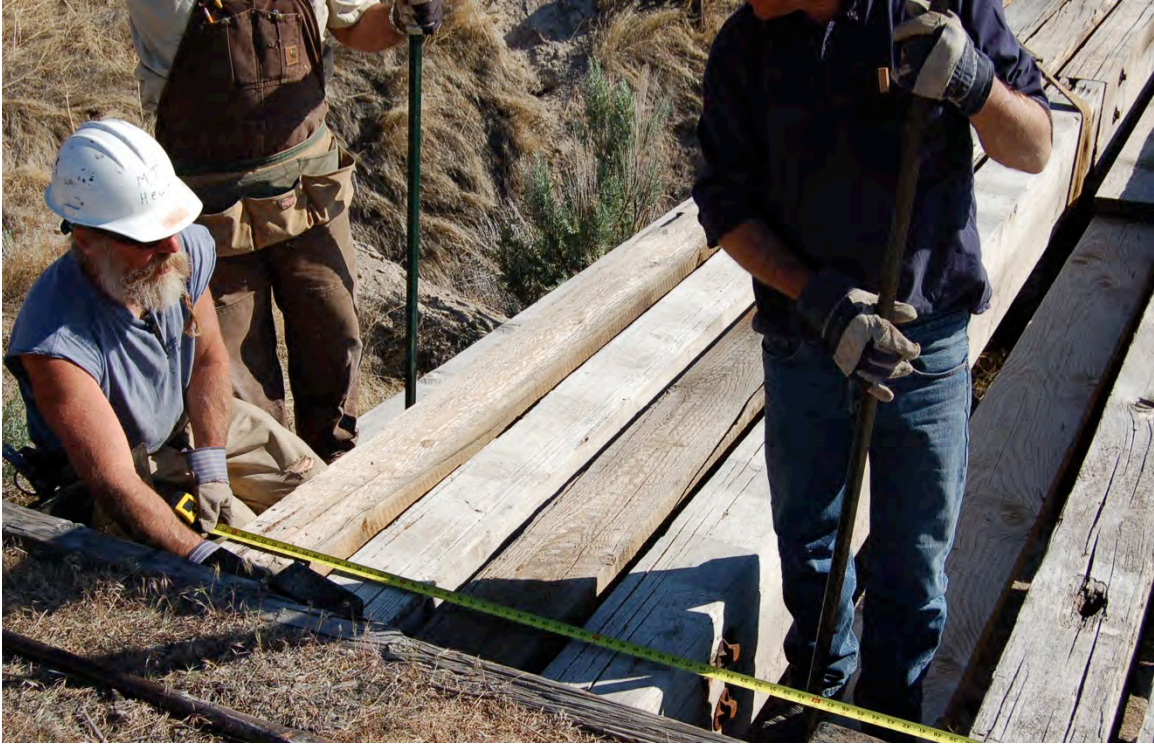
Figure 93: Adjusting the position of the assemblies to match the original.
