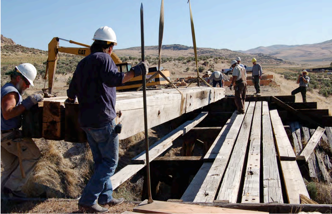
Figure 92: A stringer assembly is lowered back onto the trestle.
