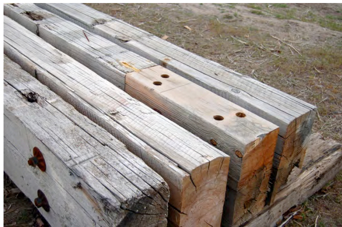
Figure 38: A dutchman repair on the third stringer from the left, Trestle #2.
