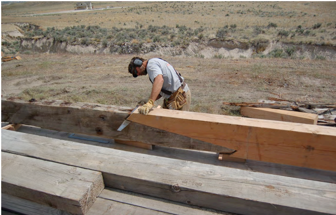
Figure 61: Adjusting the fit of a scarf joint.
