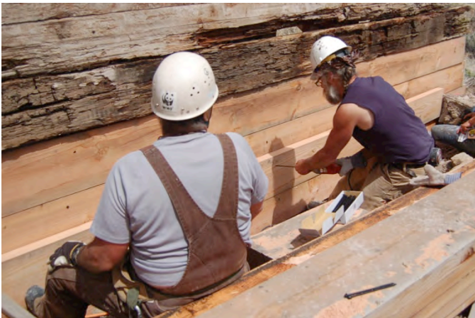
Figure 31: Installing the second layer of planking at the west bulkhead.
